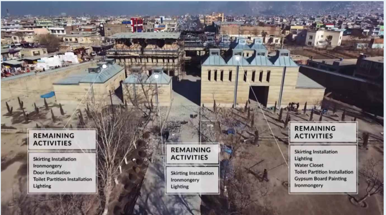
Drone image listing remaining activities.
