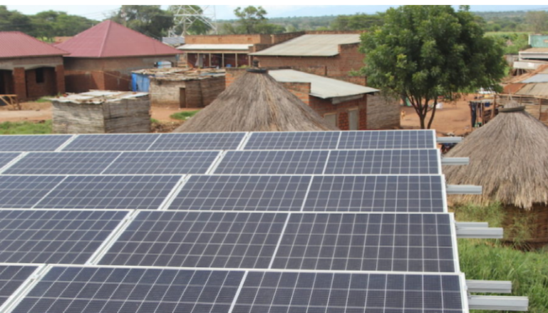
Solar panel installation in village in Uganda
